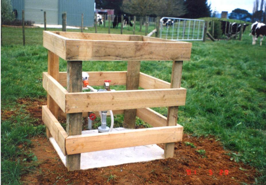
**Figure 4: An example of sanitary wellhead completion**
