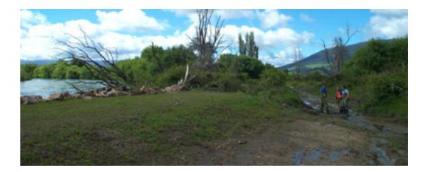
Figure 15: A low stopbank contains the Tongariro on the West side of Downs Pool. The river level is higher than ground level at the end of Awamate Rd.
