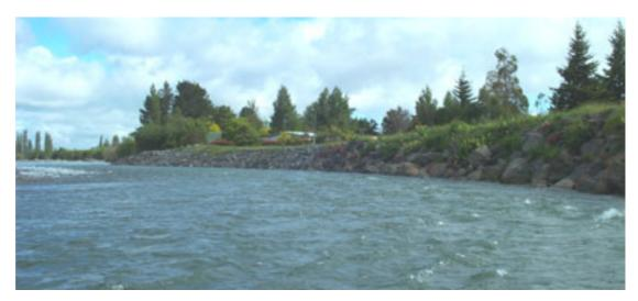
Figure 11: Rock to protect Herekiekie St Stopbank from river attack.
