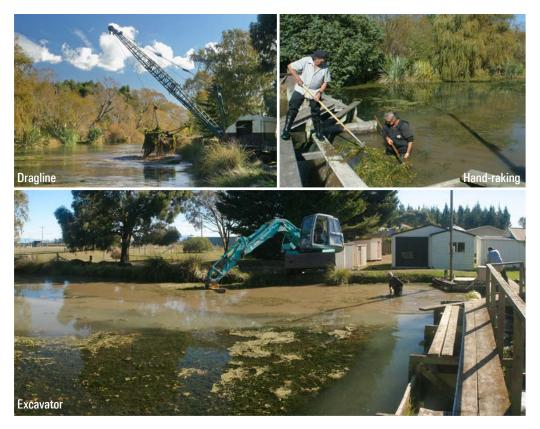
FIGURE 1 Some mechanical methods of macrophyte control used in New Zealand.
