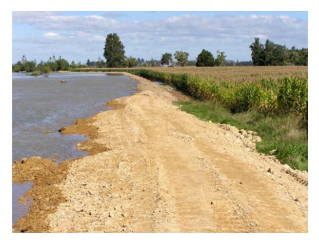
Figure 6: A newly built private stopbank adjacent to the Waikato River near Mercer (view looking south towards the old Meremere Power Station). Note the difference in elevation between the maize crop and the river level.
