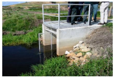
Figure 32: Flow controller, water inlet and barrier for carp trap - McLeod Morass
