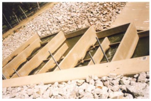
Figure 3: Fish pass on Torrumbarry Weir
