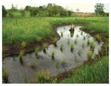
Silt traps have been constructed on all drains entering Lake Kainui. Once the native plants have established, the trap will have similar functions – and benefits – to a wetland.
