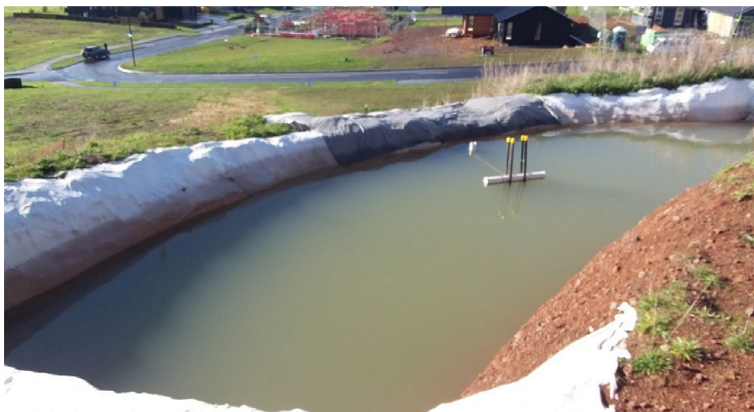
Figure 2: Sediment retention pond with 100mm clarity.
