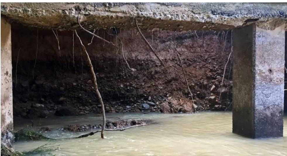
**Figure 21** Eroded bridge abutments at Waharau Bridge, April 2017 (photo credit: Ruwade Bryant/Fairfax NZ)
