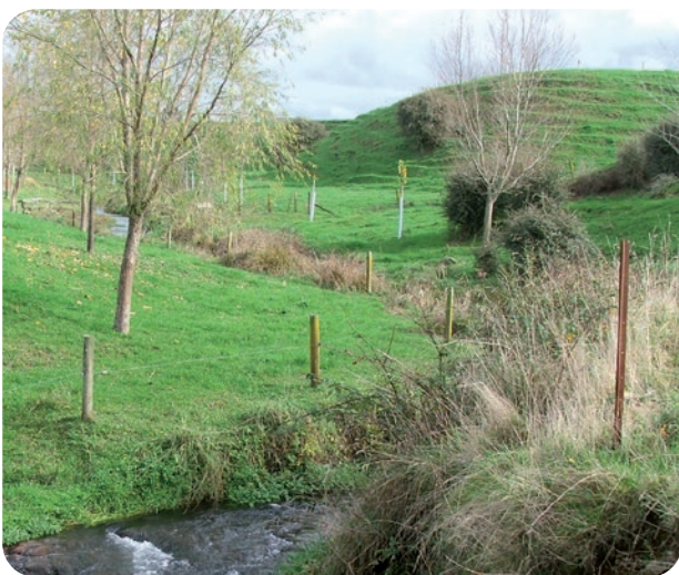
Moutere tree willow planting for stream bank stabilisation.
