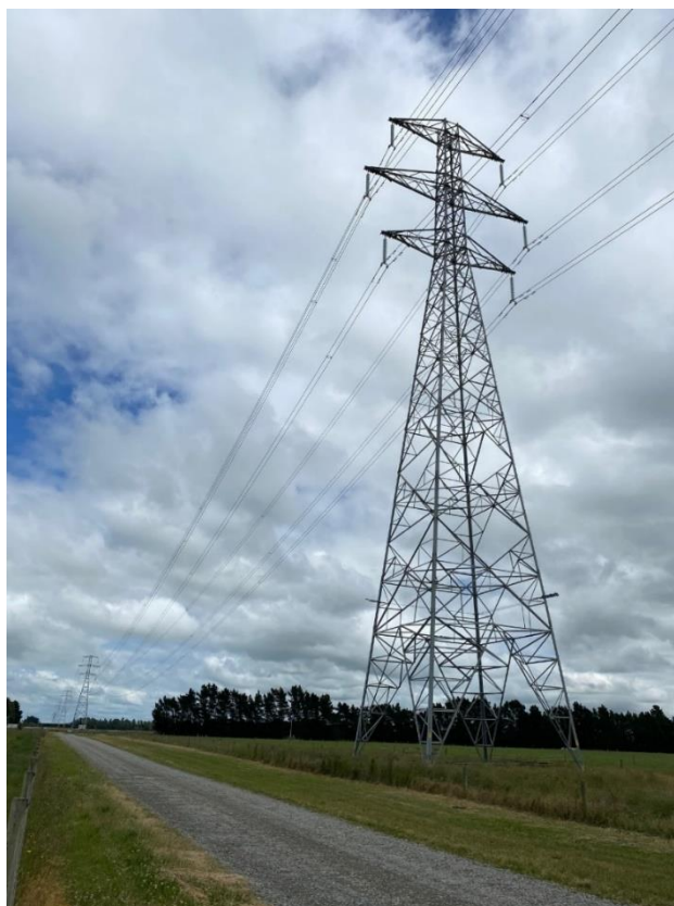
An example of overhead transmission lines - Transpower 220KV line Lincoln, Te Wai Pounamu, South Island
