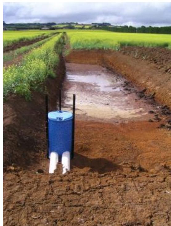
Photo 25. A silt trap with the blue snorkel in the foreground for slowly decanting the trap. A mustard cover crop is planted in the immediate paddock along with many of the paddocks in the background.
