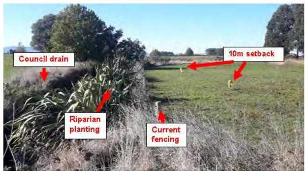
**Photo 1:** Illustration of council drain, riparian planting, current 3-4m setback and area that would be included in the setback if a 10m setback was required. The drain is able to be mechanically cleaned form outside the current fencing but could not be cleaned from outside fencing if a 10m setback was required.
