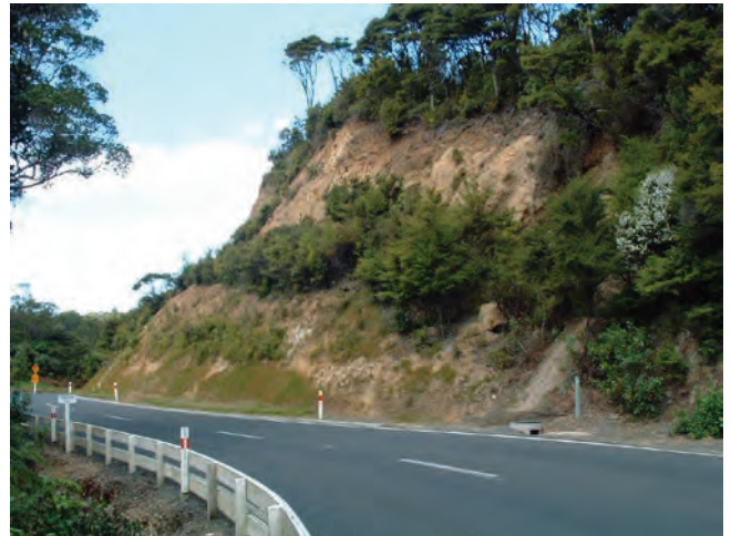
Planting road cuttings with appropriate species will assist in stabilising soil.
