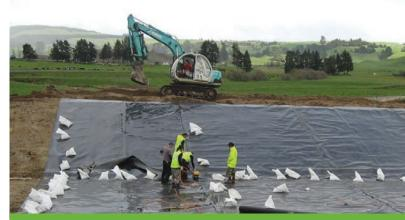
Storage pond for dairy shed effluent allowing land based effluent application at optimal times.
