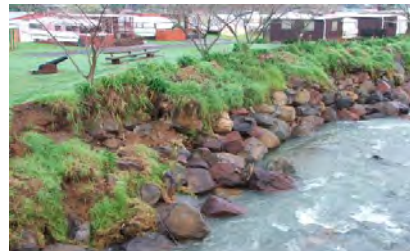
Rip rap along Te Puru stream
