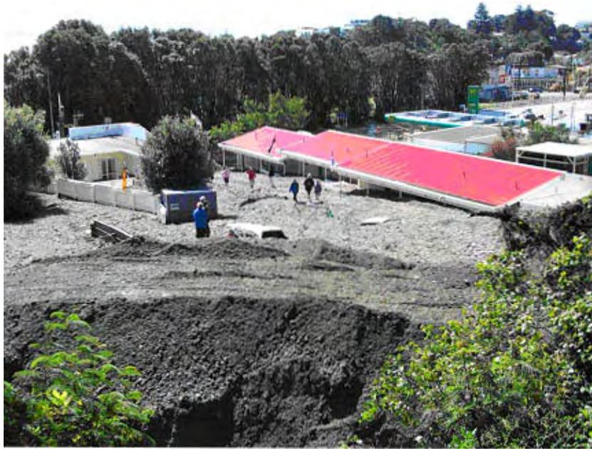
**Figure 1.3.2** Debris-flood gravel from the gully exit near Paekakariki Hill Road, north of Wellington, as a result of a storm of 3 October 2003 burying the Belvedere Motel and cars (Hancox G T, 2005).
