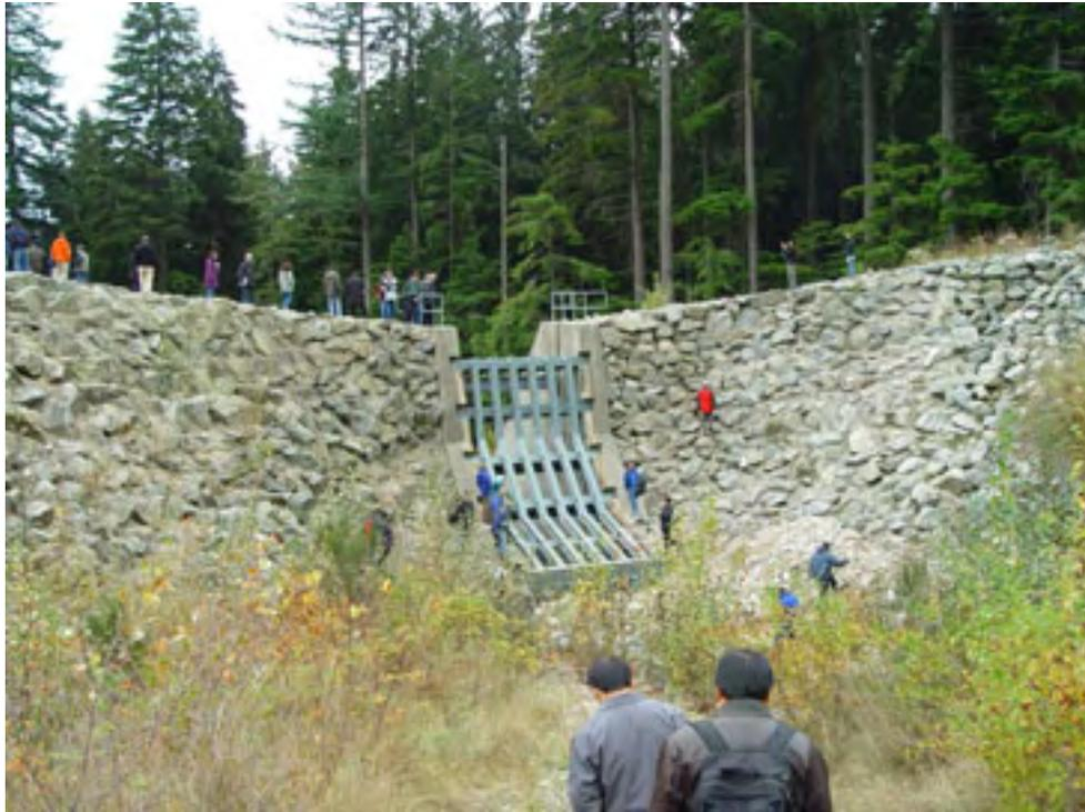
**Figure 6.0.1** A debris-retention outflow structure in a sediment-storage basin protecting a northern suburb of Vancouver, Canada. This structure is intended to safely stop events occurring about once in 500 years. To retain this capacity, the basin must be maintained relatively free of debris, and would be cleared after each significant sedimentation event even when these were not debris flows. There is a service road to access the basin for sediment removal.
