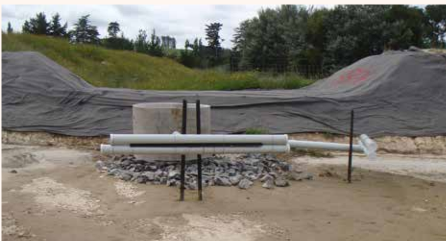
Sediment retention pond showing decant system.
