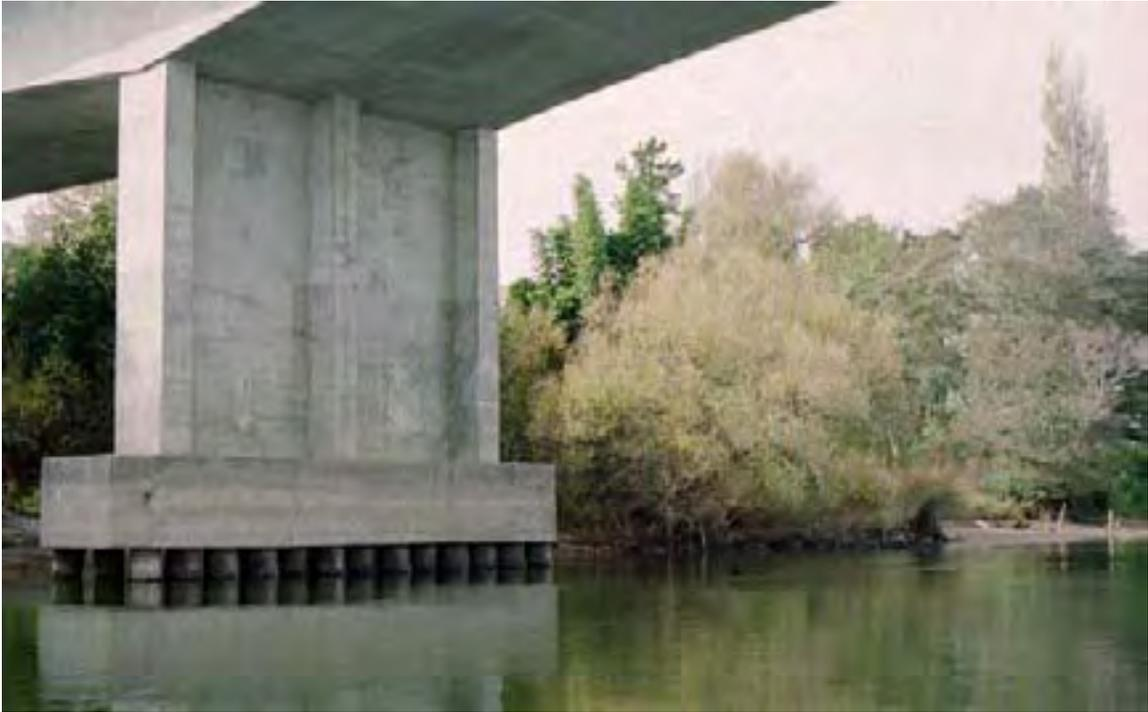
**Figure 1 Pukete Bridge showing piles exposed below the pier cap.**
