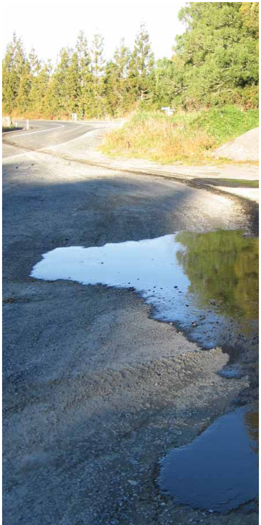
Typical spillage scene.
