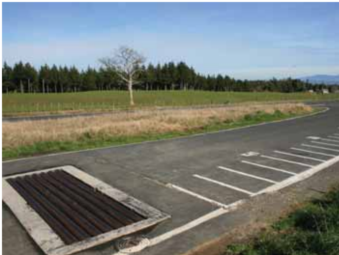
Figure 6: Stock effluent disposal facility located at Tapapa on State Highway 5 between Tirau and Rotorua.
