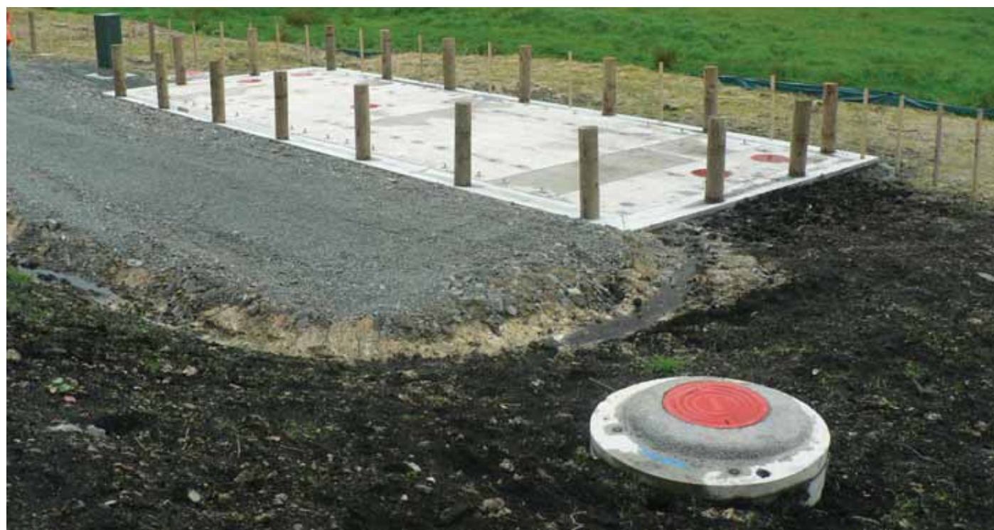
A typical effluent holding tank arrangement – Wellsford.
