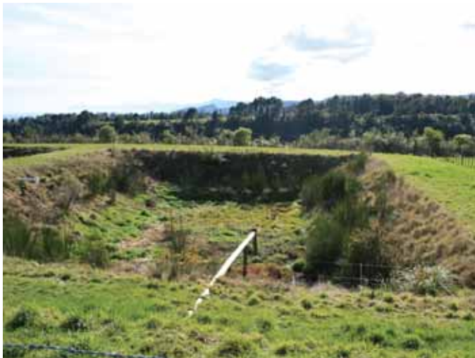
Figure 7: Settling pond at the Tapapa site.
