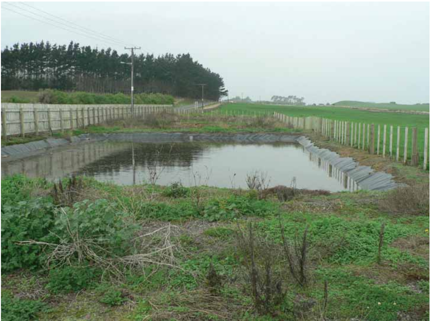
Stock effluent settling pond located on State Highway 3 near Waverly.
