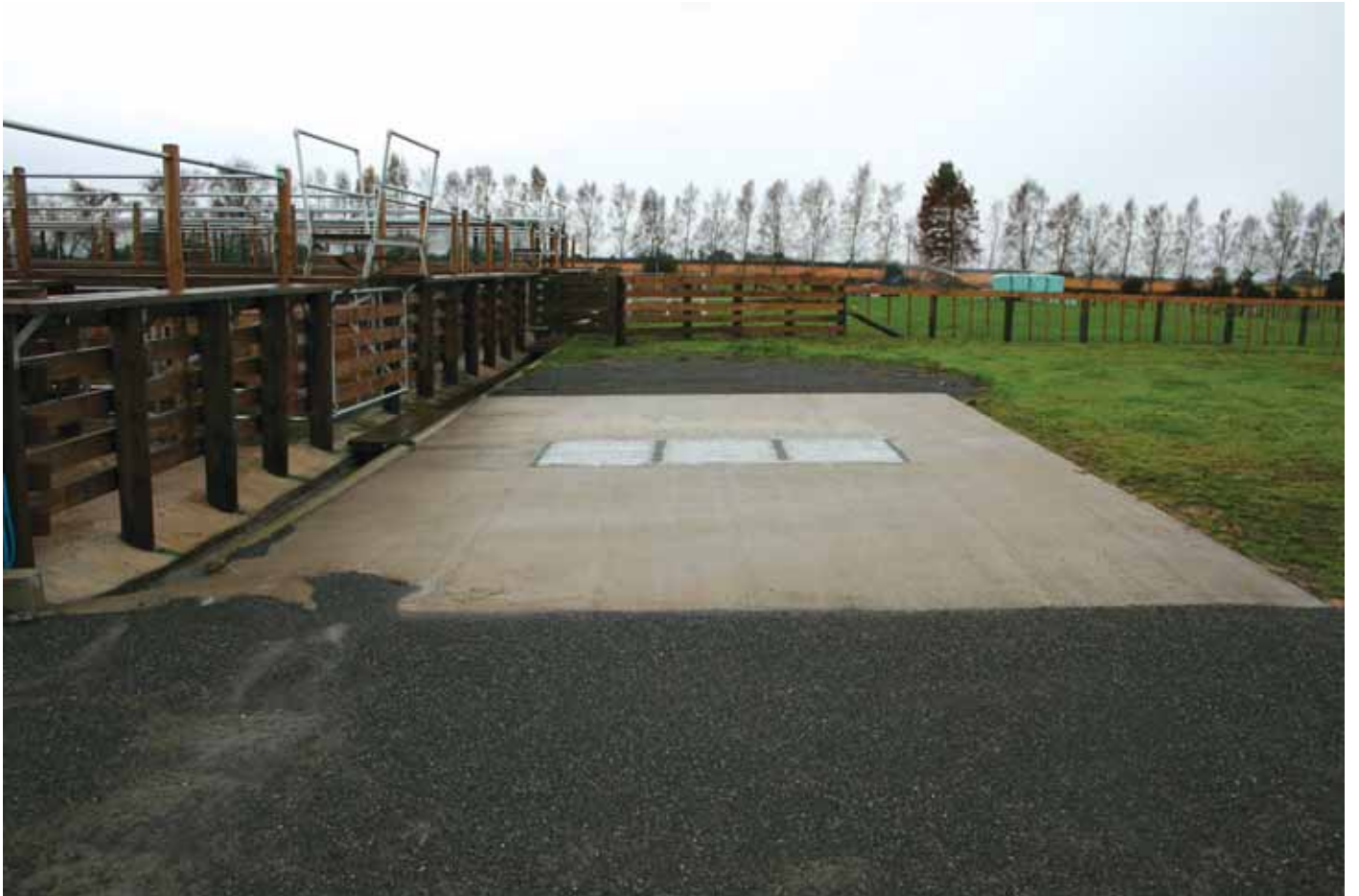
Effluent disposal facility at Matamata sale yards.
