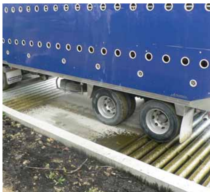
A two-grill disposal facility.
