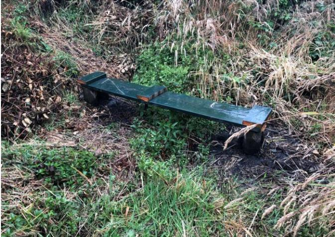
Figure 3 - Footbridge over Okaia Stream immediately below proposed crossing point in January, 2019 - note no defined channel and no flow.
