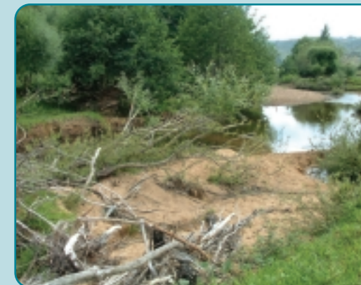
Debris and sediment blockage, Manaia River, 2003
