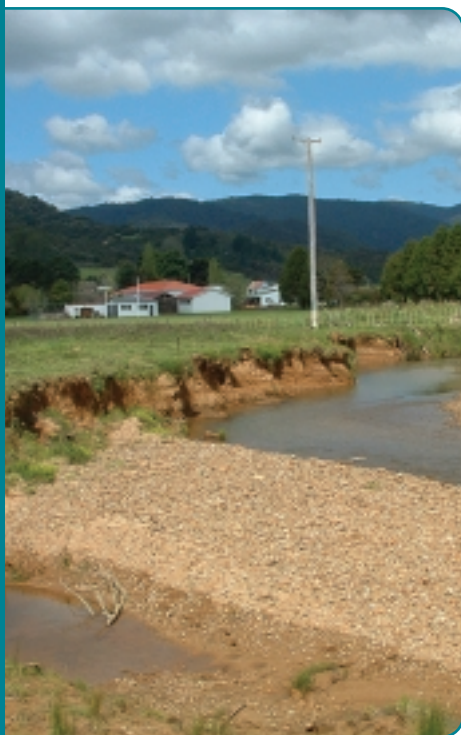
Riverbank erosion and gravel build-up, Manaia River
