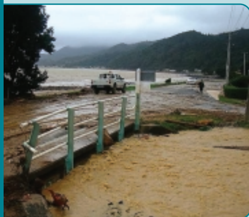
Flooding across SH25, Ngarimu Bay, 2002
